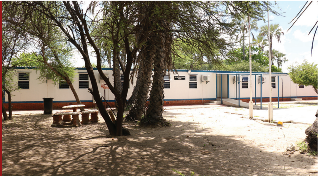
The new administration block which was constructed at a cost of P1.5 million
